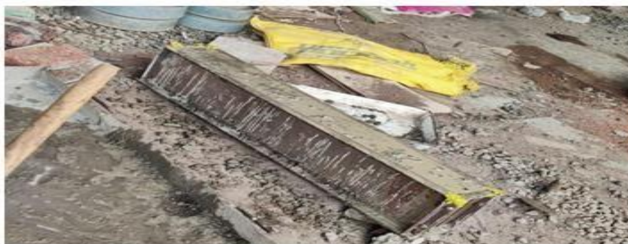
Figure No. 5.5: Casting Of Beam
